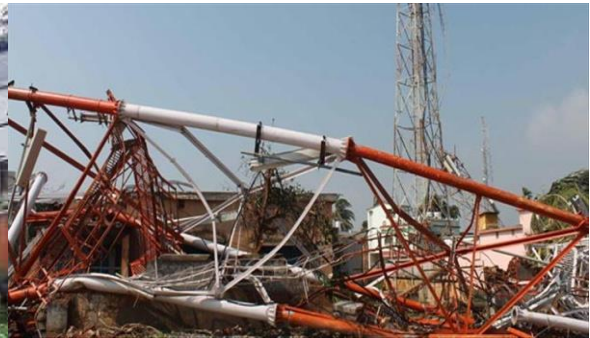
Fig.10(ii): Uprooted mobile towers in coastal AP (India)
