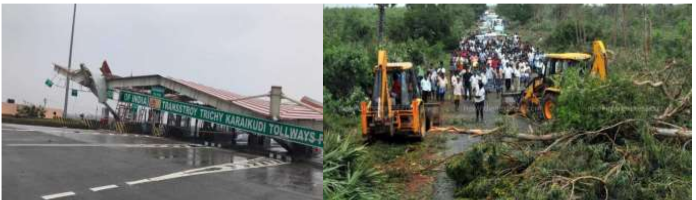
Fig.8 (d): Damaged Karaikudi Tollways and blocked roads in Tamil Nadu (The Indian Express 15.11.2018)
