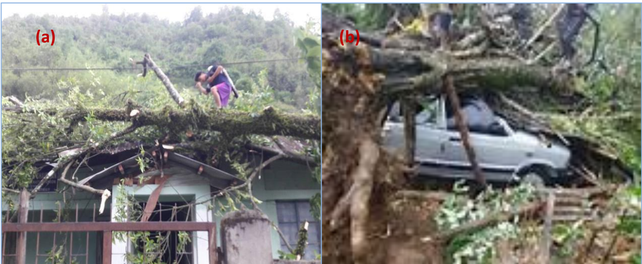
Fig. 12: (a) Damaged house in Mizoram and (b) Fallen trees (Hindustan Times, 16 May)
