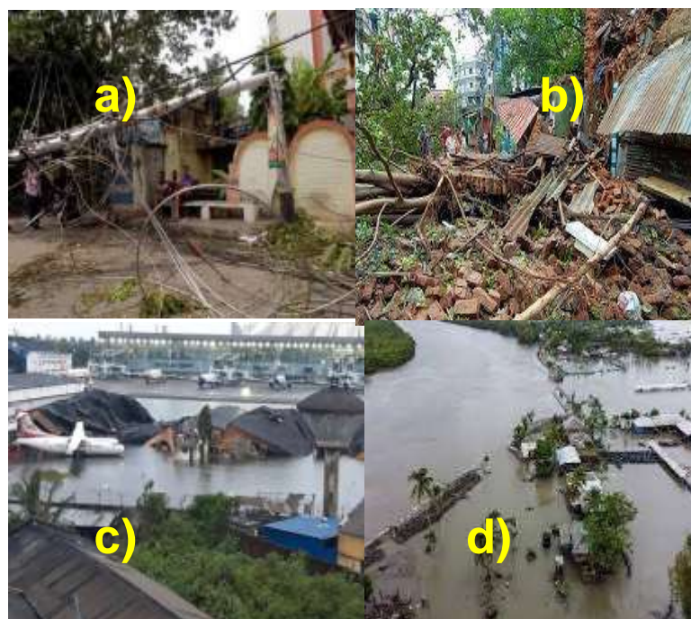
Fig. 16: (a)Hanging electric pole(The Hindu,23 rd May) (b)Flooded Kolkata Airport (NDTV,4 TH June) (c) Damaged homes (outlookindia.com,22 nd May) (d) Flooded area of West Bengal (cnn.com,22 nd May)
