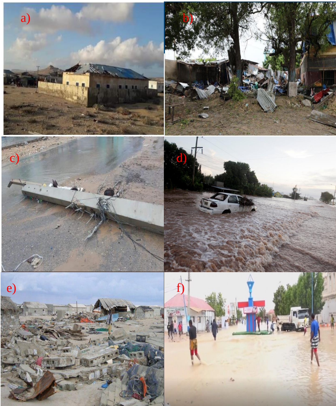
Fig. 2.8.8 (a) A house damaged by Cyclone Gati in Xaafuun district. (source: OCHA report dated 25 Nov.).(b) Damaged houses (source: https://www.aa.com.tr , dated 25 Nov.). (c) Fallen electric pole (source: from a twitter user ) . (d) Flood in Puntland’s Bari region in Somalia (source : https://newscentral.africa ,dated 25 Nov.) . (e) Gati battered Puntland coastal areas (source: https://guquddetv.com/ dated 23 Nov.) .(f) Flood havoc in the coastal town of Bosaso in northern Somalia (source: https://www.myanmaritv.com/ dated 24 Nov.)
