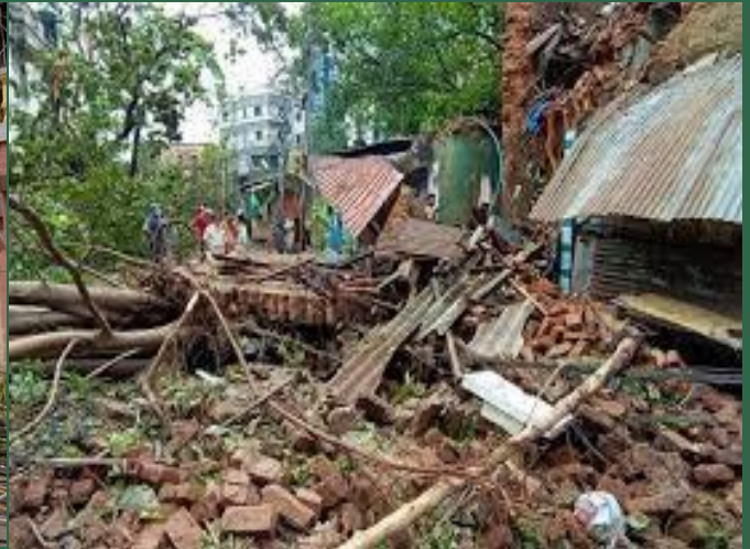
Damaged homes (outlookindia.com,22 nd May)
