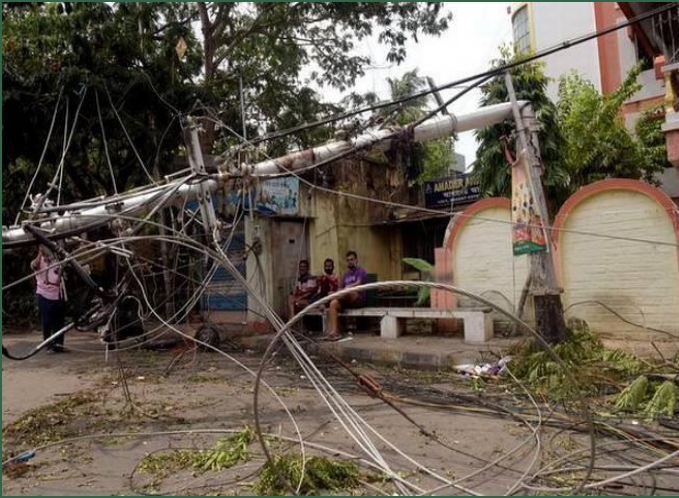
Hanging electric pole(The Hindu,23 rd May)
