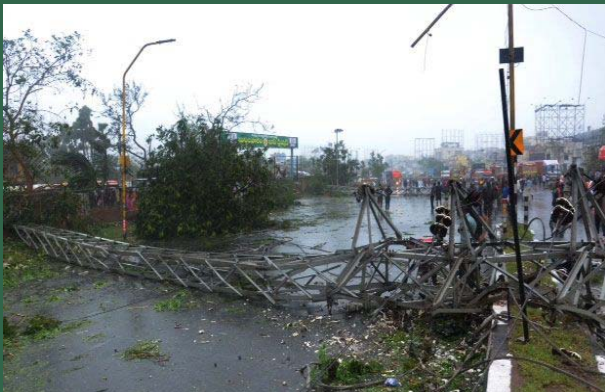
The collapsed telephone tower
