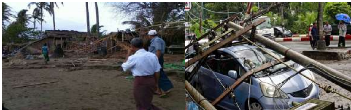
Fig.2.1.12: Damage photographs from Myanmar
