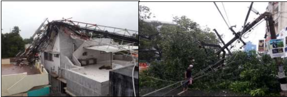
Fig. 2.9.18 (b) Damage due to gale winds over Kanyakumari (Source: M.O. Kanyakumari & IndiaToday.in, New Delhi, 30th Nov 2017)
