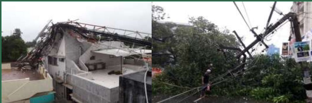
Damage due to gale winds over Kanyakumari
